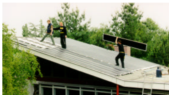
Figure 2: Installation of the first amorphous AC-modules in the Netherlands. [Photograph courtesy of Peter van der Vleuten, Free Energy Europe, The Netherlands]
